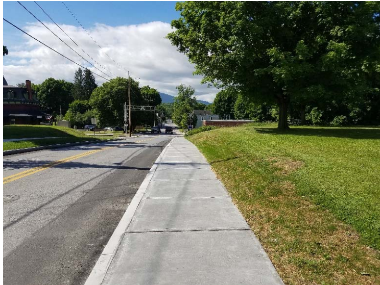
Sidewalk w/ Curb
